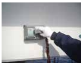
Investigation of location of reinforcing bars
