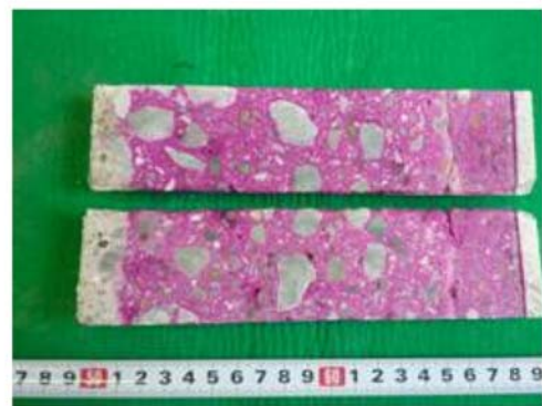
●中性化深さ測定状況
